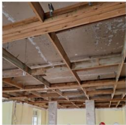
Plancher caisson bois CHU Angers
